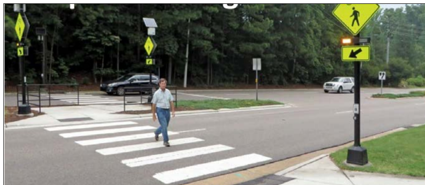
Figure 4 Pedestrian crossing beacons with a median island in the suburban area (59)
