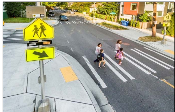
Figure 11 Curb Extension with flashing beacons for the pedestrian crossing at School Zones (92)
