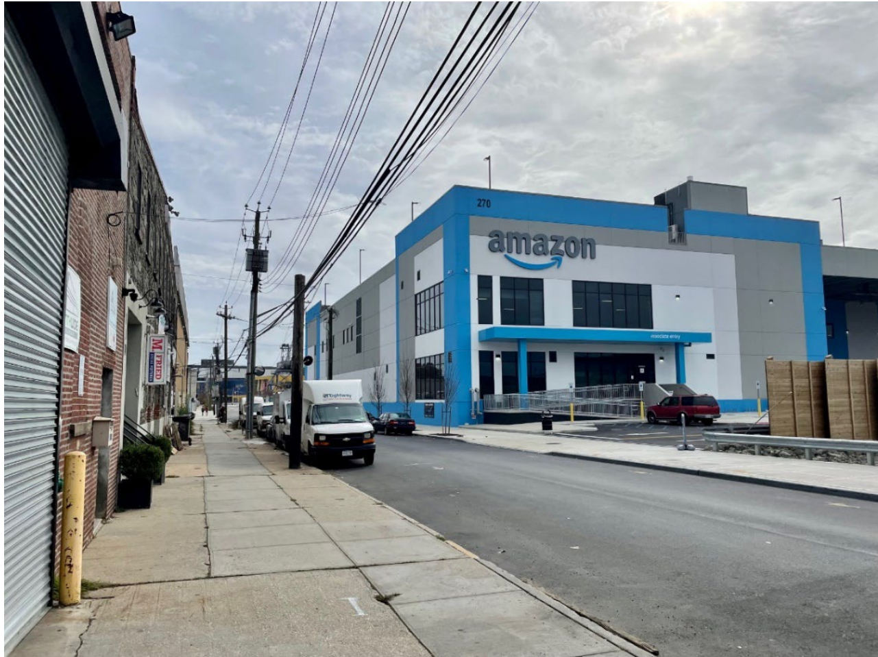
Figure 39 Multi-Story E-Commerce Delivery Center in Brooklyn
