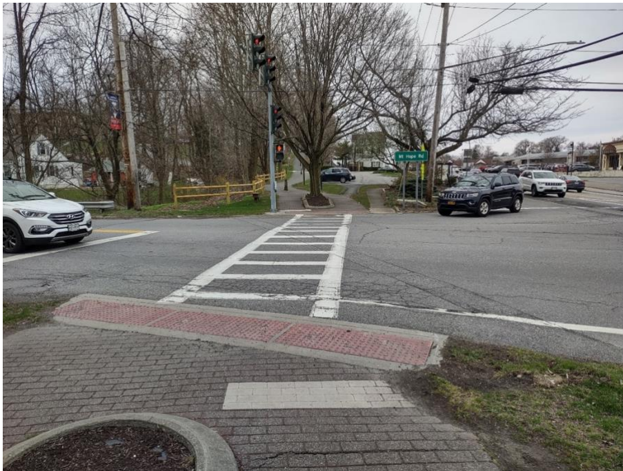
Figure 4 The length of Mt. Hope Rd Crosswalk exposes pedestrians to potential collisions. Those utilizing the Putnam trail and nearby parking have to cross this busy intersection on their way towards downtown Mahopac.
