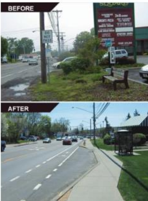
Photo of Upper Front Street in 2000 (before redesign) and 2013 (after completion of redesign). Prior to the redesign, bus passengers were required to wait in a location on the side of the road with no sidewalk access and no shelter. After the reconstruction, passengers are now able to access a new bus shelter by sidewalk, and buses can pull into a separate lane to pick up passengers. A bicycle lane has also been added to this section of Upper Front Street.
