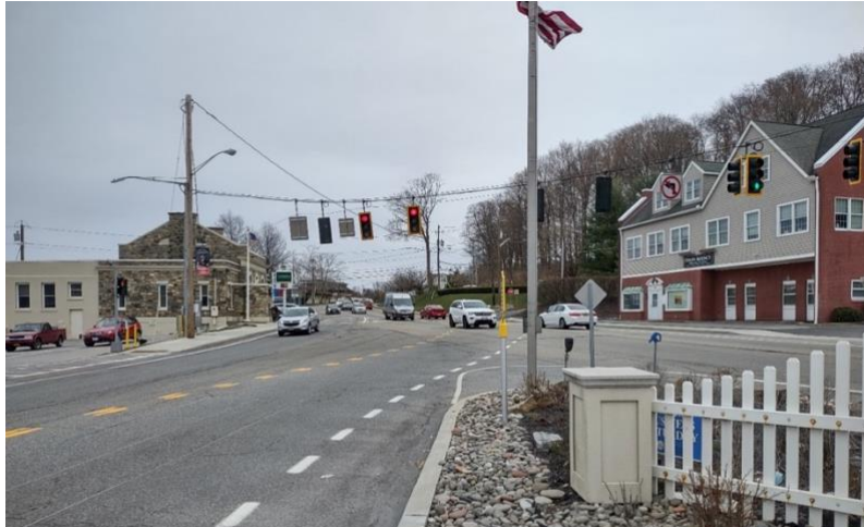
Figure 8. The current condition of Route 6N with traffic in both directions. The merge with Route 6 has been a site of several traffic collisions. Source: POET.
