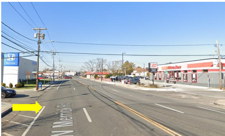
Figure 9. Streetview of Merrick Road at Montgomery Street showing lack of crosswalk markings and signage at this intersection. Source: Google.
