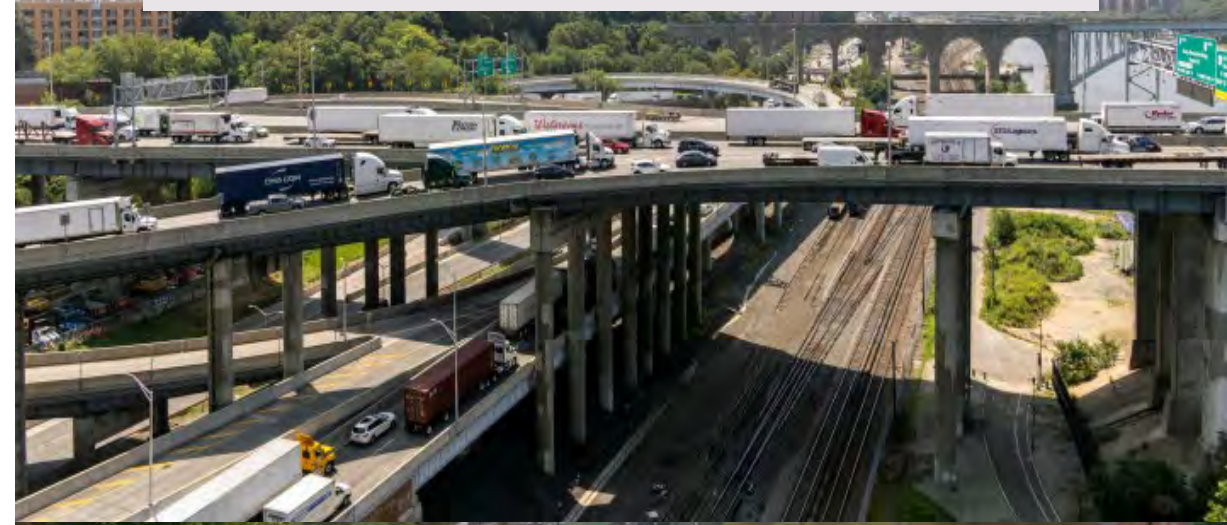
Macombs Avenue over the Cross Bronx Expressway
