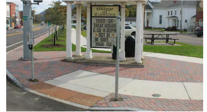
ADA ramps, Village of Canisteo
