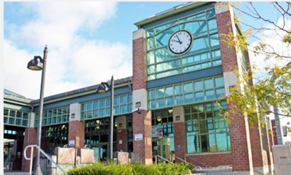
LIRR Hempstead Station
