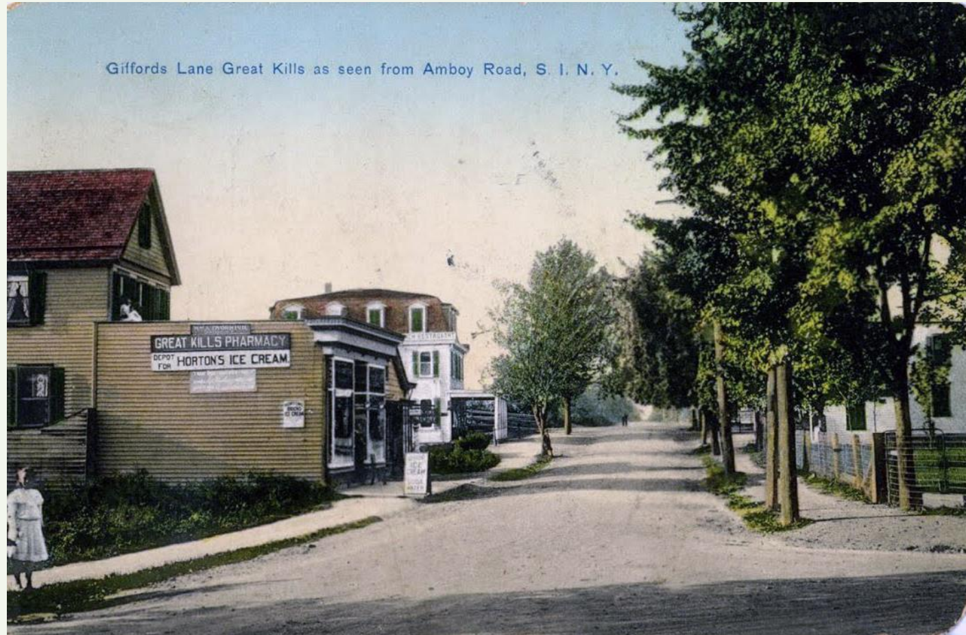
Gifford's Lane as seen from Amboy Road (Historic Image v/s Modern Day Image)
