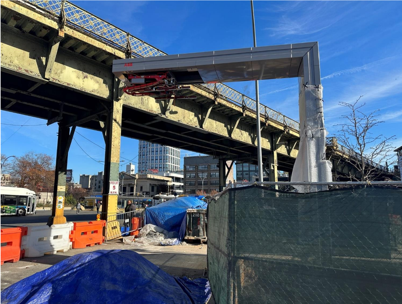
Williamsburg Bridge Plaza – Pantograph Mast
