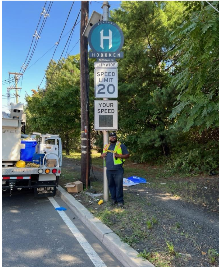
Speed radar feedback signs installed at 8 gateway locations
