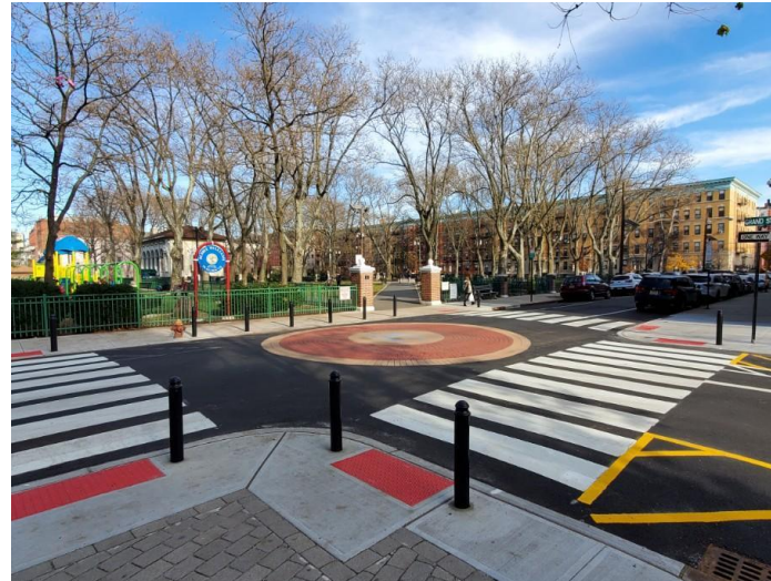
Raised intersection with high visibility crosswalks installed as part of Hoboken's annual roadway resurfacing program outside school and park at 9 th Street & Grand Street
