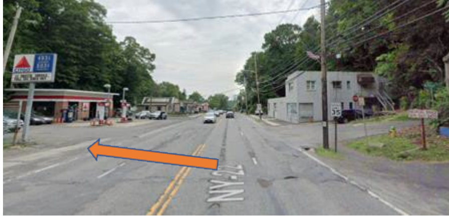
Photo depicting poor sidewalk conditions and the area for a proposed midblock crossing. Source: NYMTC-POET Images from Site Visit November 21, 2022.
