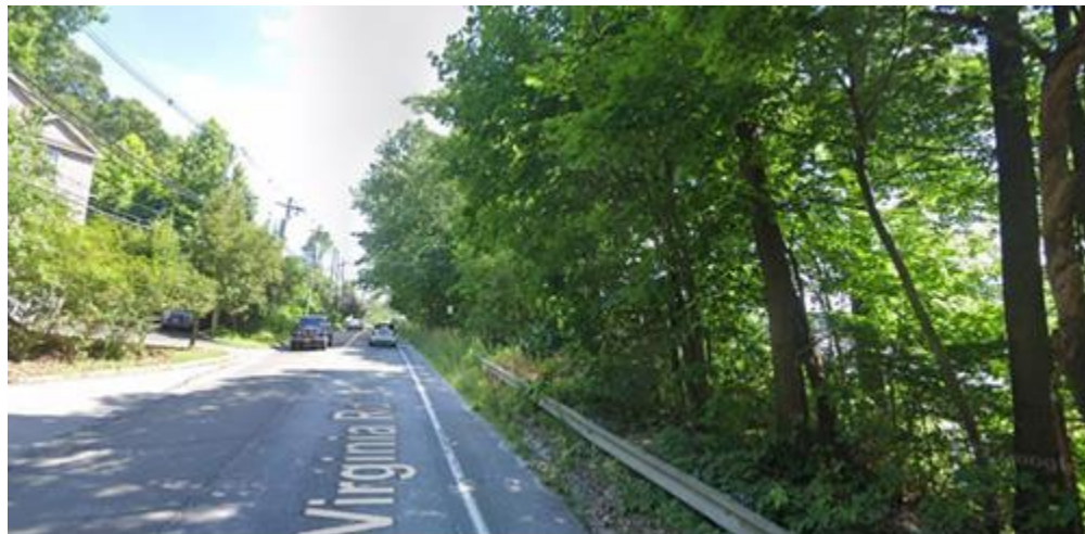
Photo depicting the lack of sidewalk network along Virginia Road. Source: NYMTC-POET Images from Site Visit November 21, 2022.
