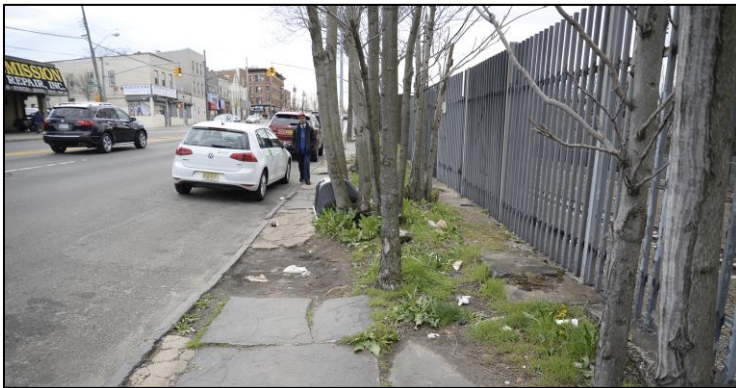
Sidewalks with adequate width but internal obstructions restrict movement
