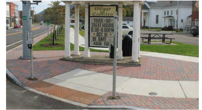
ADA ramps, Village of Canisteo
